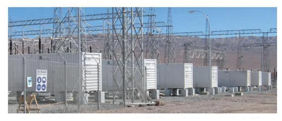
Figure 3.3. Li-ion battery supplying up to 12 MW of power at Los Andes substation in Chile
