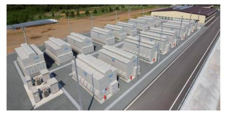
Figure 3.10. NaS battery unit – 34 MW in Japan
