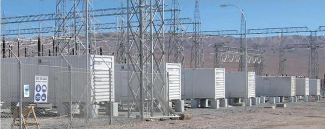
Figure 3.3. Li-ion battery supplying up to 12 MW of power at Los Andes substation in Chile
