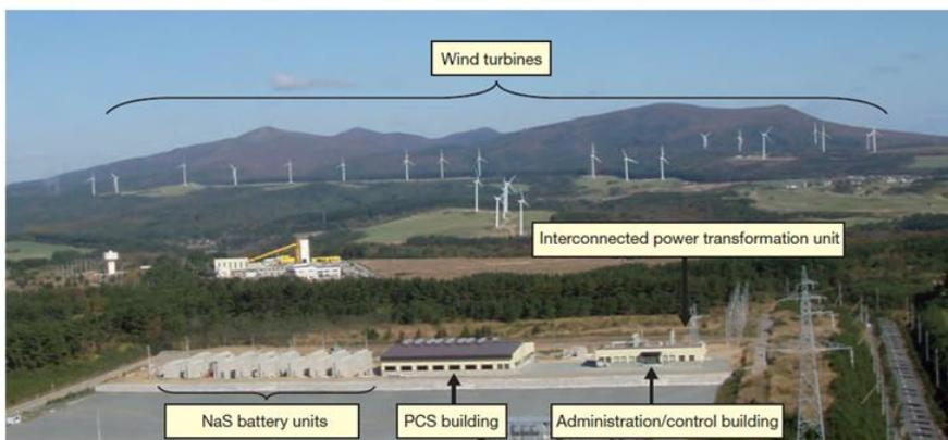
Figure 3.9. General view of the Futamata wind power plant in Japan
